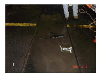
This shows an example of what we were dealing with, at the throat of the tunnel we were at 27' below sea level with sea water seeping in around a lot of these joints. As we removed the asphalt to repair the joint water was constantly seeping in. We would attempt to seal the joint the best we could with an injection sealant process then fill the patch with Aquaphalt.
