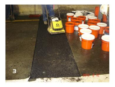
We placed the Aquaphalt in 2 lifts to make sure it didn't settle too much with the heavy traffic volume on Interstate 664. In one instance when we came in the next night, one of the patches did settle about 34" so I tried putting a skim patch on top of what we did the night before doubting that it would adhere and stay in place. Not only did it stay in place there was water still seeping out of this patch. This was approximately 3 years ago and it is still in place.
