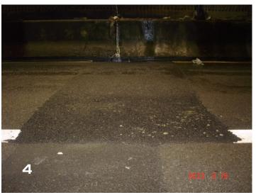
This was a pothole that was approx. 10" deep, down to the concrete below. Massive amount of sea water running out of it right in the wheel path of the right lane. Filled it with Aquaphalt to safe up the lane until we did the joint repair in this location. Aquaphalt stayed in place until the repair was performed.
