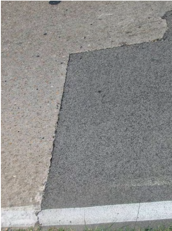
Material has maintained a uniform profile, very little to no pushing or shoving and no rutting
