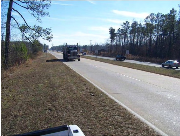
Figure 3, US Route 60 @ Bottoms Bridge
