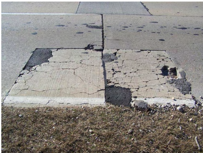
Figure 1, Evaluation site on US Route 60 West at Bottoms Bridge.
