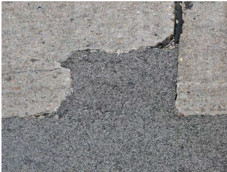
Material is in-place, stable and shows no signs of cracking
