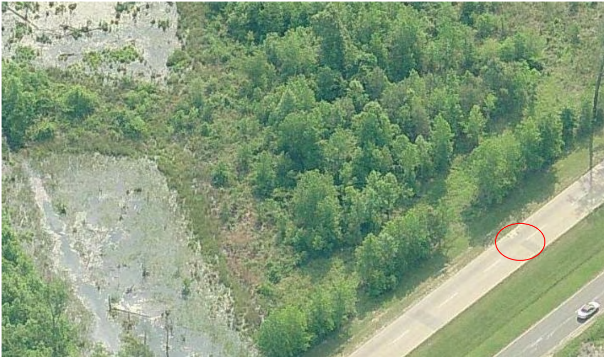
Figure 2, Aerial View of evaluation site
